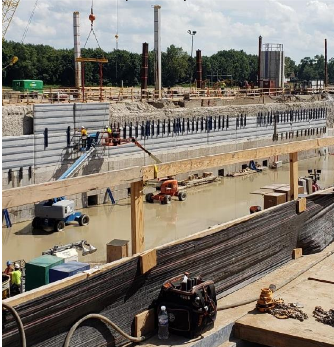
Vertical concrete pre-cast panel installation
