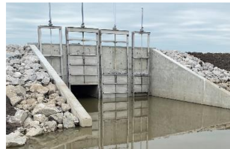
Clarence Cannon Water Control Structure MVS
